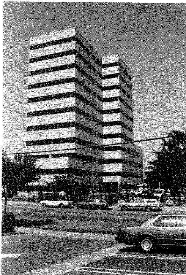
Medical building featuring exterior walls of shop manufactured perlite portland cement fiber-reinforced plaster panels.
