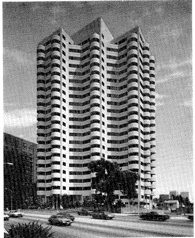
The walls on this luxury high rise condominium consist of flat and curved steel stud framed elements that were shop assembled and plastered with perlite portland cement fiber-reinforced plaster.
