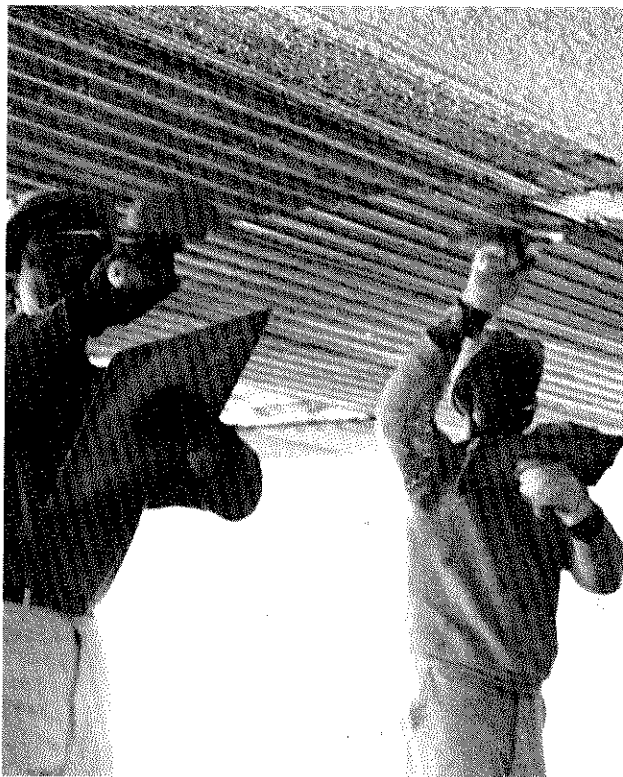
Lightweight perlite gypsum plaster provides an ideal base coat plaster for interior walls and ceilings.
